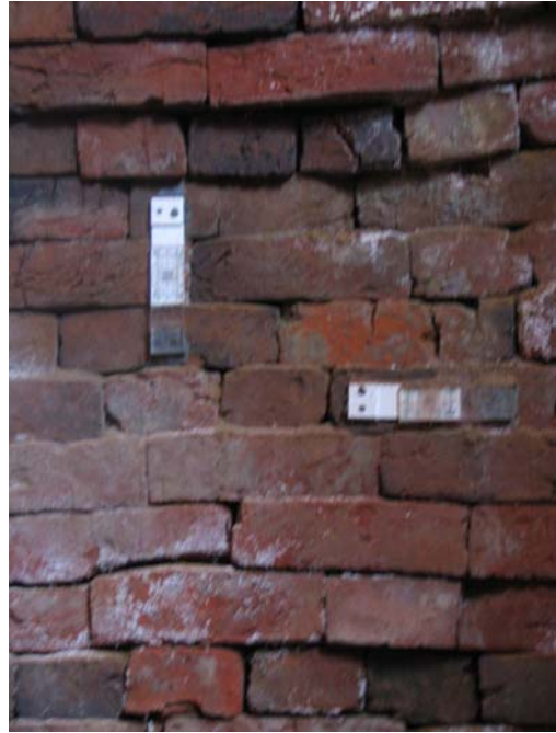
Crack monitoring of a collapsing portion of the ice well wall.
