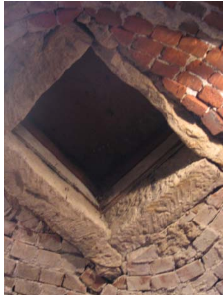
View looking up at the original street level "hatch."
