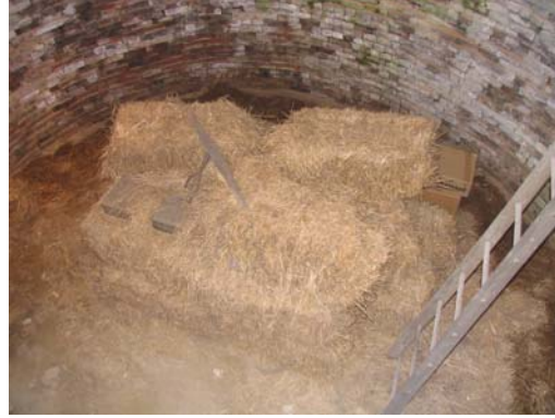
A view looking inside the ice well.
